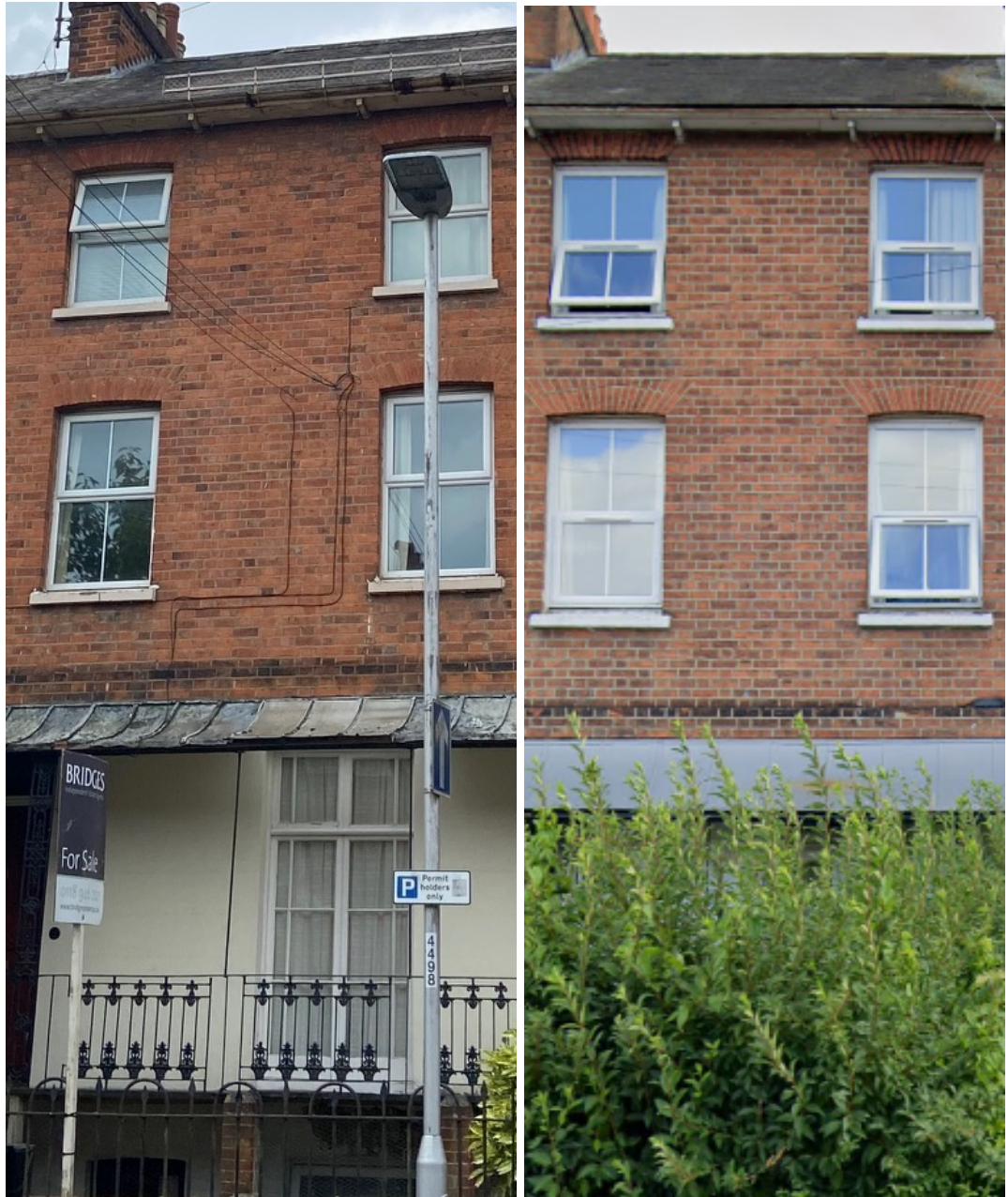
Poor quality replacement non-sash style uPVC windows elsewhere within Jesse Terrace
